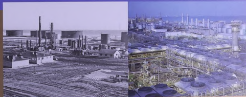
Saudi Aramco's first refinery at Ras Tanura was a 3,000-bpd "tea kettle" facility. Today, Ras Tanura's refining capacity is more than 500,000 bpd.
