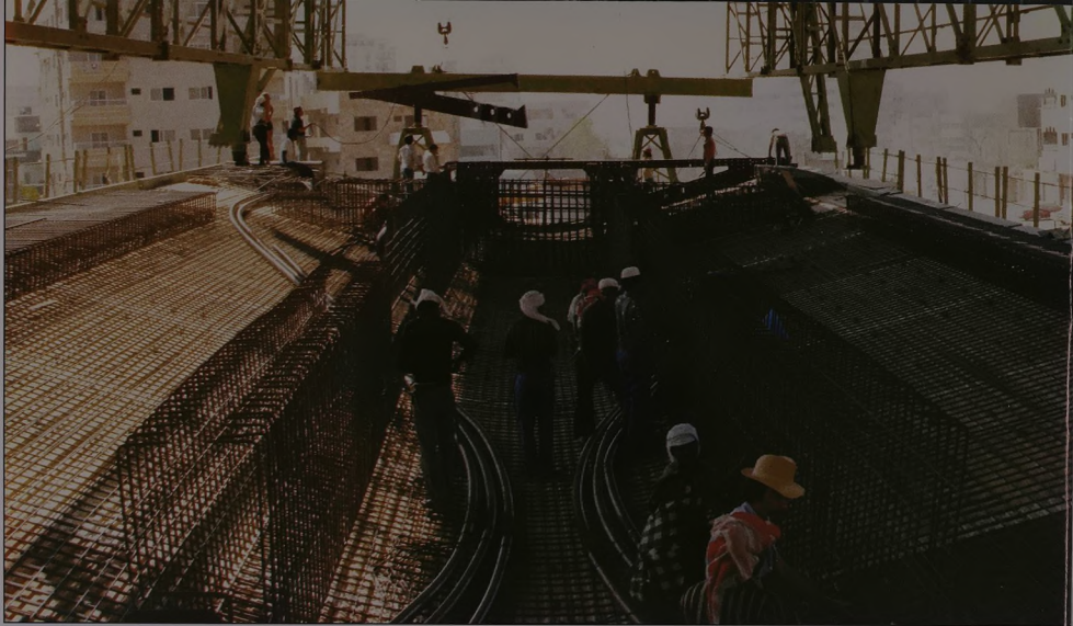
Building the Outer Ring Road, Riyadh
