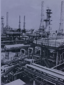
The 62 million dollar oil refinery at Basra in Southern Iraq built by Czechoslovakia, with an annual capacity of 3.3 million m tons.
