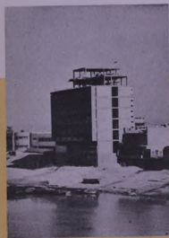
The new Maternity Hospital under construction: 7 floors, 400 beds.
