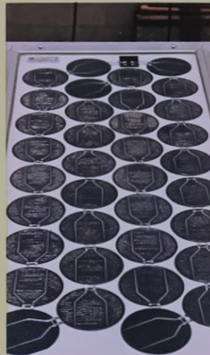
Photovoltaic Panels mounted on Solar House Roof
