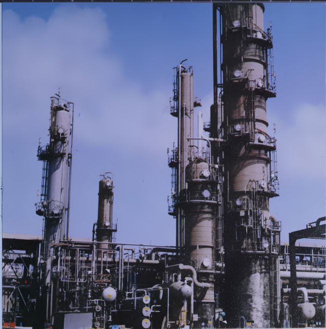
A Close-up of one of the two Trains in the Plant
