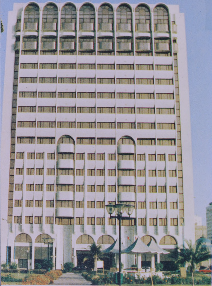
ADGAS Main Office in Abu Dhabi
