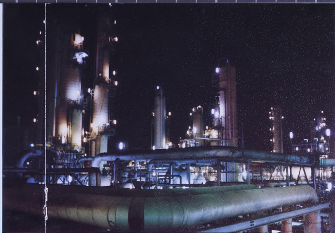
A General View of the LNG Plant by Night
