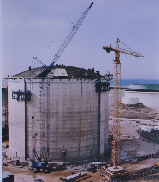
One of the Tanks under Construction
