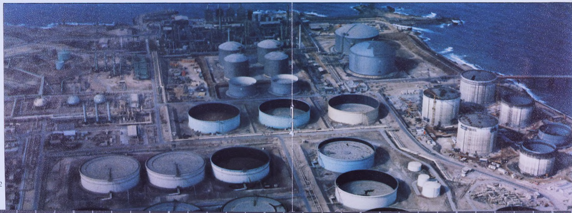
Gas Feedstock Is Supplied to ADGAS Plant by ADMA-OPCO
