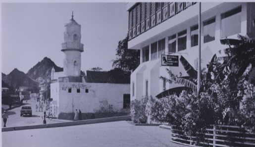
The National and Grindlays Bank in the old town of Muscat
