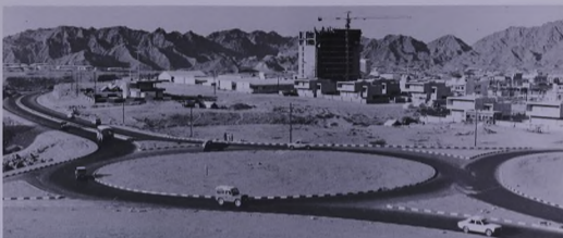
Part of dual-carriageway section through the Ruwi valley of the Mutrah to United Arab Emirates road.
