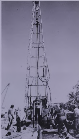
Drilling for water
