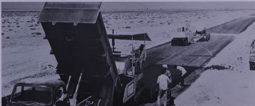
Constructing the new Salalah-Taqah road
