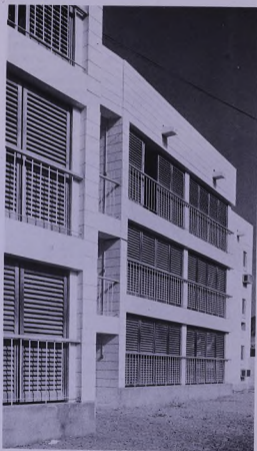
Staff accommodation, Ruwi Hospital
