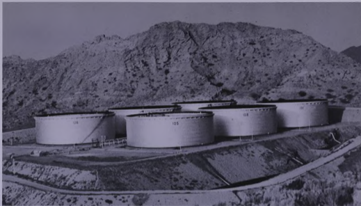
Crude oil storage tanks at Mina al Fahal
