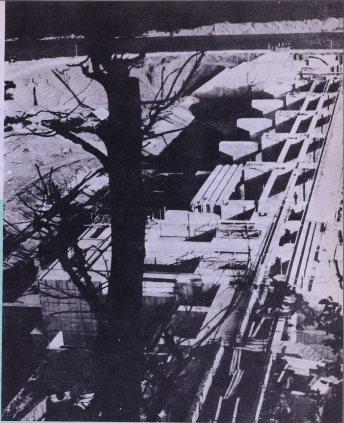
Another view of the Tarik dam, Gilan province
