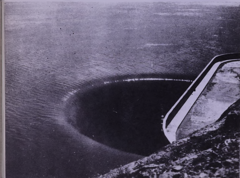
Shaft spillway of Empress Farah Pahlavi Dam, Gilan Province
