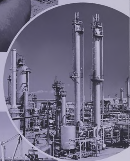
This stabilizer removes fuel gas and LP Gas from naphtha.
