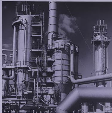
This is one of two crude distillation units at the Ras Tanura refinery.
