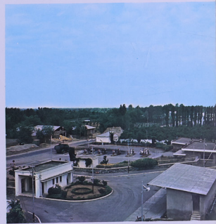
Oil storage at Chalous
