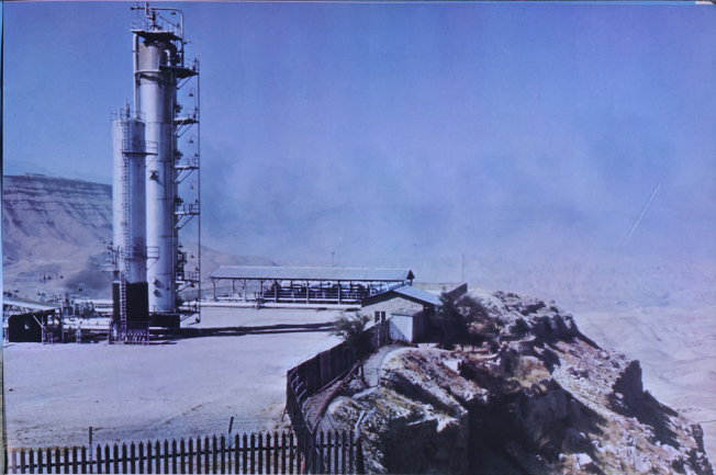
Production Unit No. 1 at Gachsaran.
