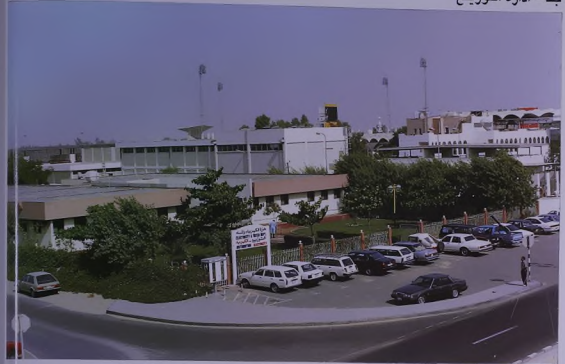
Electricity Distribution Department - Sharjah
