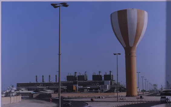
Layyah Elevated Tank opposite to Layyah Station
