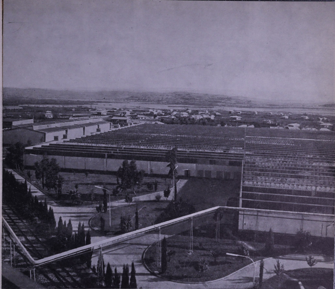
General view of Shahi No. 2 textile mill
