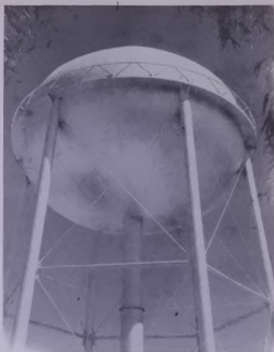
The new Water Supply Project.
