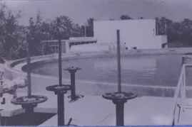
Purification pool of the Water Supply Project.
