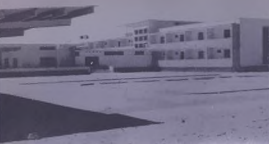
The Rest House in Karbala — completed this year.
