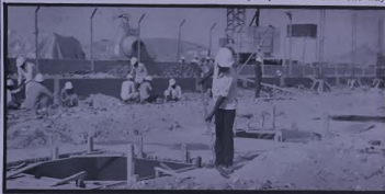
* Construction of a new wing began on 5th April.
