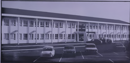
In 1977 a third two storey wing was added to the main office block at Mina al-Fahal.
