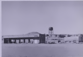
At the new 'Udhailiyah base for the Ghawar Field are these garage, water and shop facilities.
