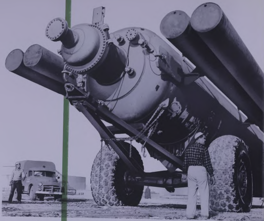
Giant 10-foot tires help transport the 182-ton reactor column for the catalytic desulfurization unit at the Ras Tanura refinery.
