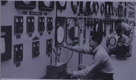
Rodney Martin, 'Ali Isma'il, J. E. Nolan check the Ras Tanura boiler controls.
