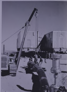
This auxiliary pumping unit at Wari'ah will help boost the delivery of oil to Tapline facilities.
