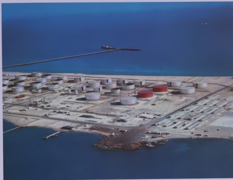
Saudi Arab contractors helped construct the new storage tanks (red) at the Ras Tanura terminal.
