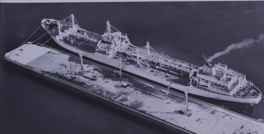
The improved south pier of Aramco's Persian Gulf terminal can accommodate most supertankers.
