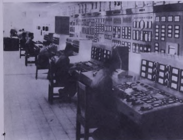
Control equipment, managed by expert technicians The workshop of the central electric plant where different kinds of spare parts are manufactured
