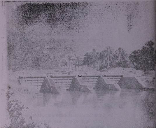
Main Canal fronte ( after its dredging )
