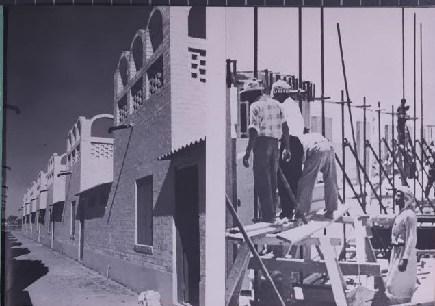
Low cost workers housing. These houses in the West Baghdad Housing Development were constructed by the Development Board. They contain two rooms, kitchen, store room, courtyard, sanitary facilities and shower and have a sleeping roof for the hot season.
