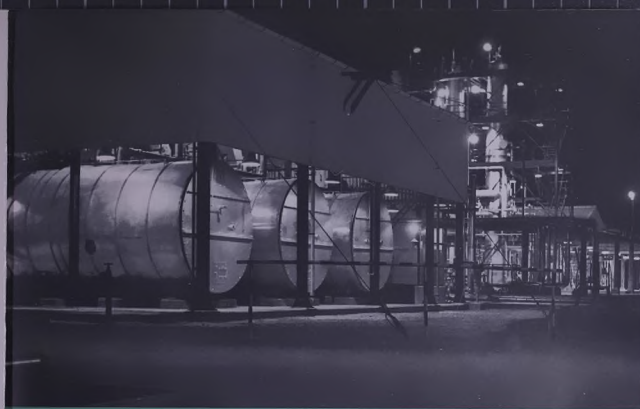
Qaiyarah Bitumen Refinery. Boiler House, with Topping Unit in background.
