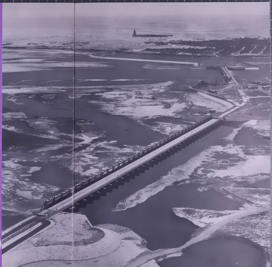
The Tigris Spring Flood was halted here for the first time in 1916. Greatest single accomplishment to date of the Development Programme is the Tharthar Flood Control Works. The Samarrah Barrage (background) diverts the Tigris flood waters through the Tharthar Regulator (foreground) into the 64 kilometer long Tharthar flood channel and the Tharthar Depression. In the distant background the Army Mosque, famous monument of the period of the Abbasid caliphs.
