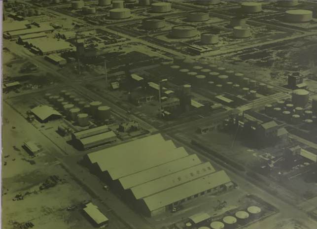
Modern Iraq: partial view of the Daura Refinery built by the Iraq Government to produce petroleum products for the domestic market from Iraq oil.
