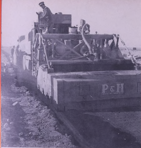
Road construction is a vital part of the Development Programme.
