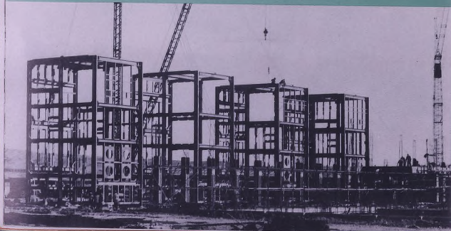
Dibs Power Station The Framework of the 4 boilers October 1957.
