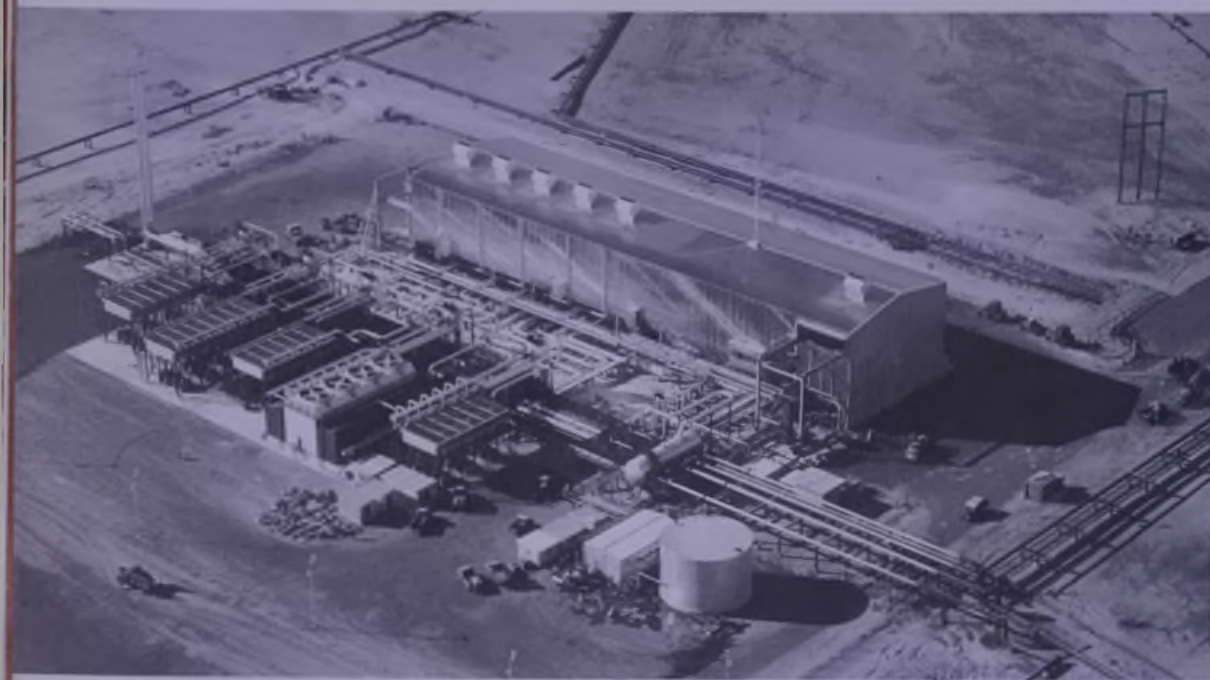
The new gas injection plant built at 'Ain Dar can compress and put back underground 200 million cubic feet of gas daily.
