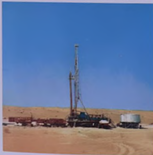
A new mobile structure drill working in the desert.
