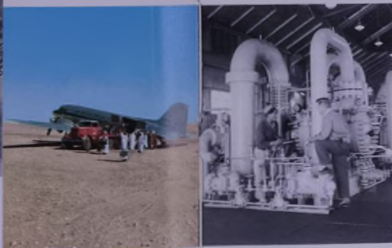
New centrifugal compressors in the Abqaiq Gas Injection Plant.
