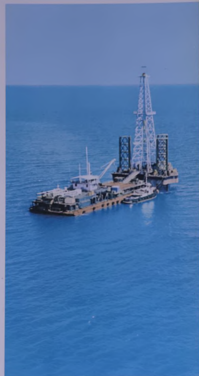
The mobile drilling platform works with the barge 'Queen Mary' (left) offshore at Manifa.
