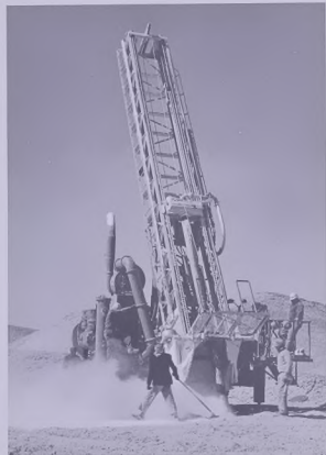
As part of the program to increase Ghawar field production, a special drill bores holes for new pipeline supports.
