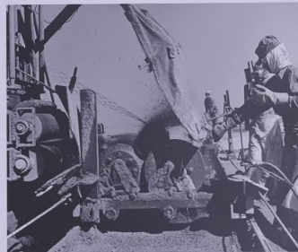
New pipe receives a protective coating before installation.
