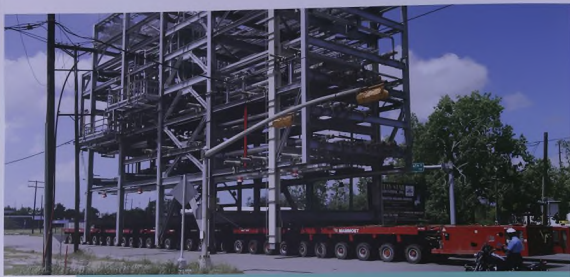
Above: A component for the expansion of the Motiva refinery in the United States is moved to the plant.
