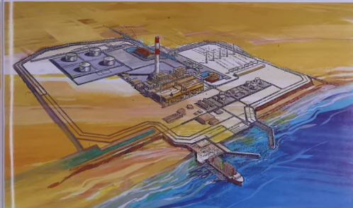
THE BIRD'S - EYE VIEW OF QURAYYAH POWER STATION (2 x 600 M/W)
