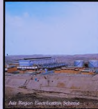
Ain Region Electrification Scheme
