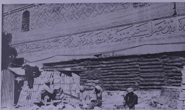
Restoration of the damaged facades
