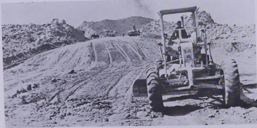
Building & paving roads
