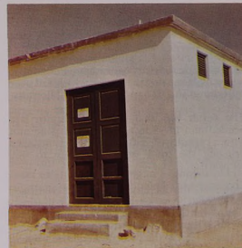
Manama Central Distribution Sub Station.
