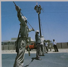
Overhead Lines Construction
