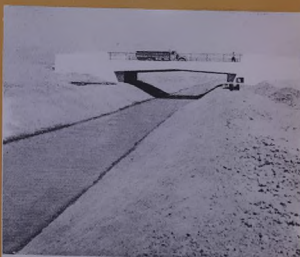
The water flowing in the Army Canal. One of the bridges constructed on the Canal is seen in the picture.
