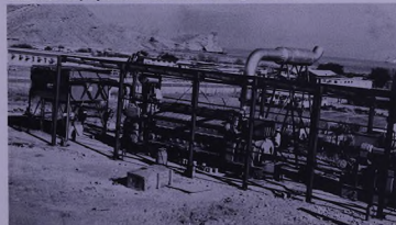
Installation of the generators nearing completion.
