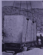
Supply Department positioning one of the new generators.
