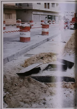
■ Re-construction of Sewerage in Palace Avenue - Manama...
