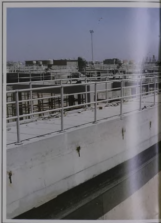
■ Expansion of Tubli Sewage Effluent Treatment Plant...
