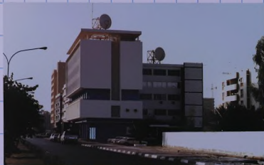
Thanks to the oil money, Abu Dhabi has flourished into a cosmopolitan city. Picture shows ADMA-OPCO's Main Office Building
