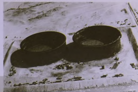
Tankage under construction
