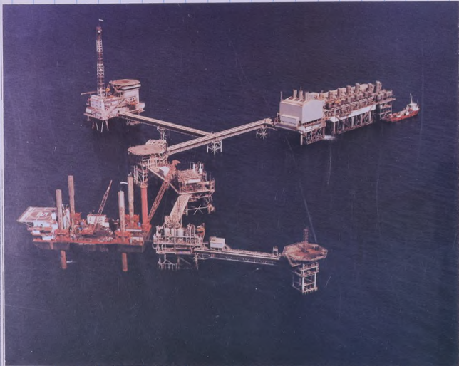
Umm Shaif Supercomplex
