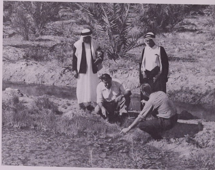
An Aramco representative explains drainage survey to officials in Qatif.
