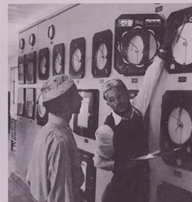
A Saudi explains control panel of the stabilizer in Abqaiq.
