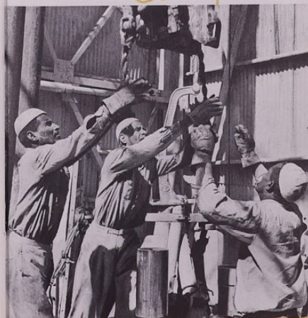
A Saudi crew prepares to attach "elevator" to hoist up another length of drilling pipe.
