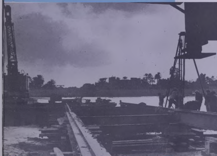
General view of the bridge site.
