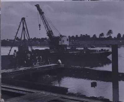
Another view of the bridge site showing the floats which were used for securing the old pontoon bridge before it was demolished.
