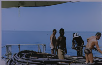
Laying the cable for marine seismic survey
