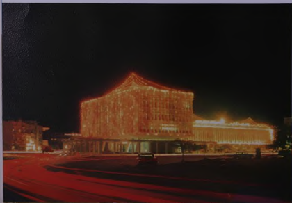
KNPC Main Office building
