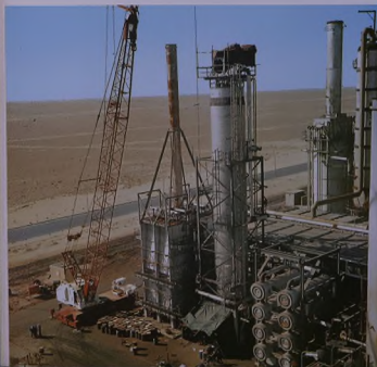
Catalyst change for the Isomax reactor
