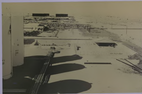
New TEL facilities in foreground and new 1,500,000 bbls/storage in background; two of the major capital additions to the Refinery during 1969
