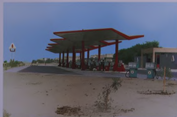
Adilyah filling station — one of the new installations constructed in 1969
