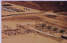
Switchyards/substations, such as the one built in 1977 at Abqaiq, at top, will be located at all generating plants and at Dhahran, Ras Tanura, and Khursaniyah. Transmission lines will branch out from the switchyards/substations to provide power to load centers with lesser energy demands such as GOSP's, refineries, residential areas and industrial plants; also completed during 1977 is the switchyard/substation built adjacent to Aramco's Sewerage Treatment Plant, above, at Qurayyah on the Gulf, at right is a section of the Jubail switchyard.
