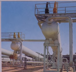
Gas/crude oil separators at a gathering centre
