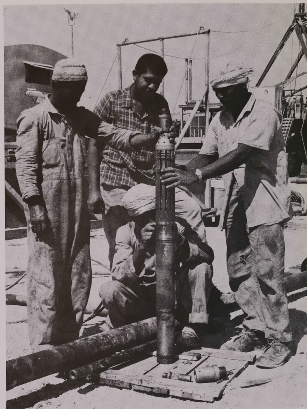
Preparation on sub-surface well safety equipment
