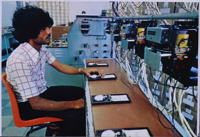
Testing meters for accuracy before installation at Consumers premises
