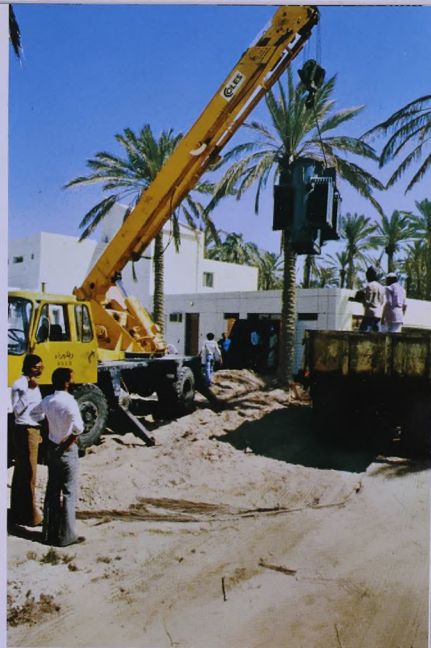
Installing a transformer at a new development
