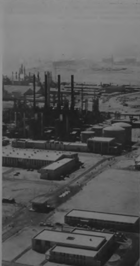
Qatar's ethylene plant
