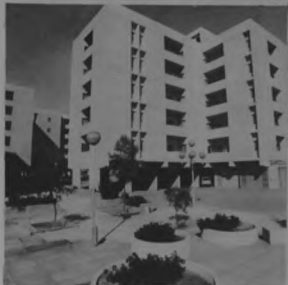
Flats for employees of Qatar Petrochemical Company
