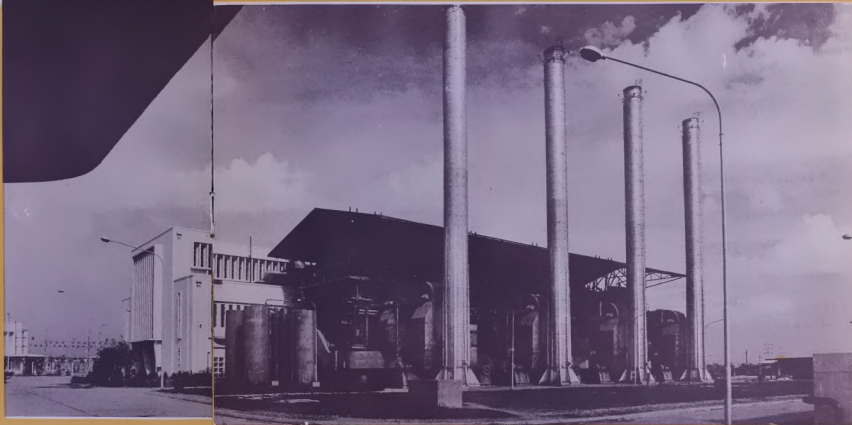
A general view of the installations of the National Electricity Services' Power House
