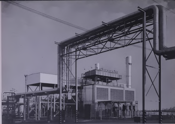
New LPG plant in Abqaiq processes and conserves 55,000,000 cubic feet of gases daily.
