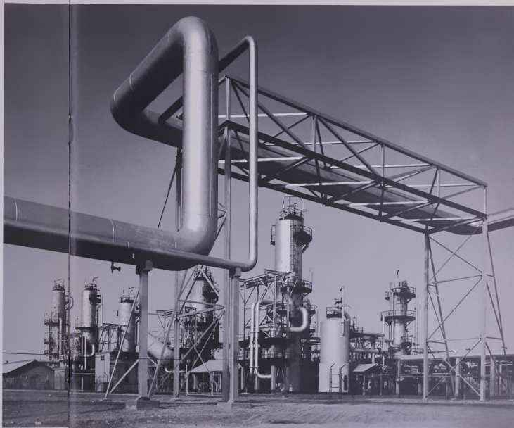
Poisonous gases are removed from crude oil by stabilizer in Abqaiq.
