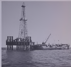
New drilling tender operates offshore.
