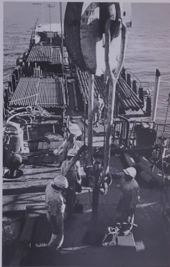
Offshore drilling crew inserts drill pipe.
