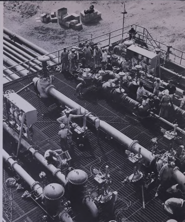
New blender fills special market needs by mixing crudes, refined products.
