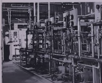
New electro-dialysis unit purifies brackish Dhahran water for drinking.
