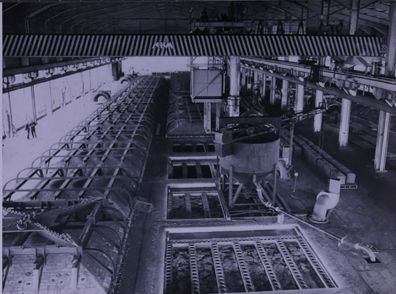
Panoramic view of Kiln 2 from the south.
