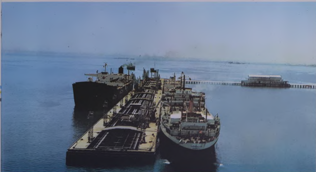
GENERAL VIEW OF THE NORTH PIER
