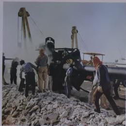
LAYING THE PIPELINE THAT WILL CARRY GAS TO SHUAIBA
