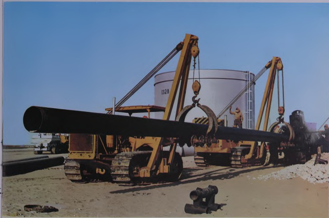
LAYING THE PIPELINE THAT WILL CARRY GAS TO SHUAIBA
