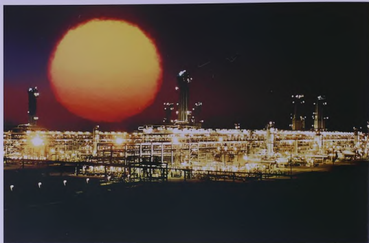
Ju'aymah Gas Plant facilities at night.
