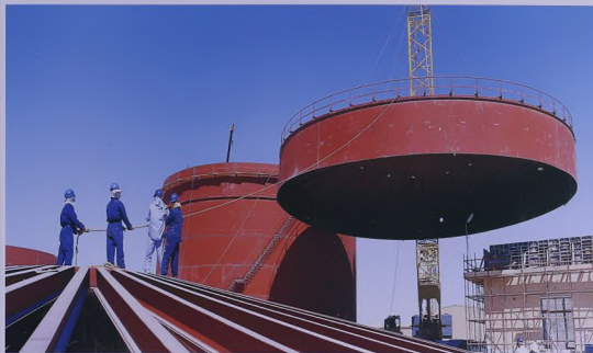
Storage tanks being assembled at Hawiyah Gas Plant. Below, a new propane surge vessel at Ju'aymah that will serve industries in Jubail.
