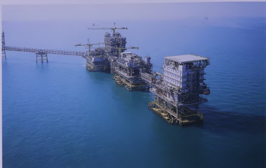
A gas-oil separation plant in the Gulf. Offshore facilities like this one are being linked to the corporate network by satellite.
