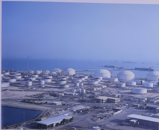
Part of Ras Tanura's storage tank farm, where the movements of crude oil and products were fully automated.
