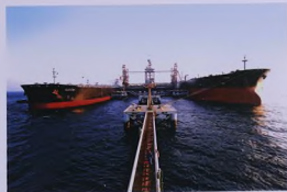
Saudi Aramco has marine terminals on the Arabian Gulf capable of handling the world's largest supertankers. The company maintains a fleet of helicopters and airplanes to ferry people and supplies to and from remote locations and offshore facilities and marine units.
