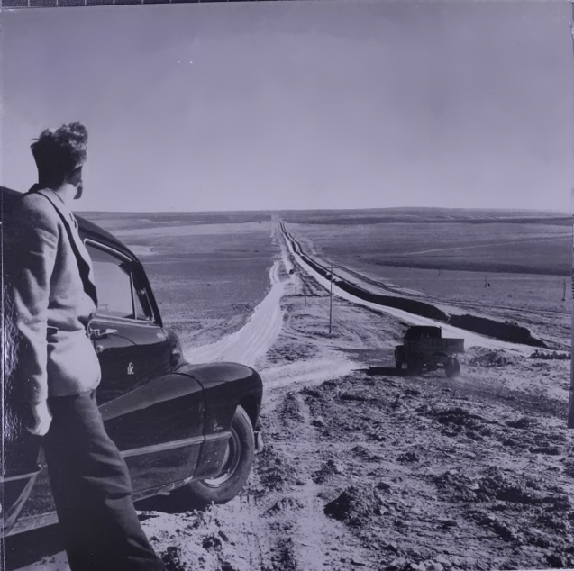
Typical of the terrain where the new 30-inch pipeline threads through rock and sand from Kirkuk to the Mediterranean
