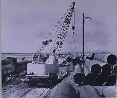
Scenes during the construction of the Kirkuk-Baniyas 30-inch pipeline
