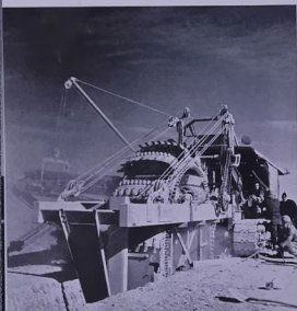
Left: a Buckeye Ditcher cuts part of the 556-mile 4 x 5-foot trench. Right: 30-inch pipe takes up a 15' bend like wax; pipe ends are bevelled before welding; a Mighly Anty, with trailer stowed, awaits its next 65-ton load of 30-inch pipe
