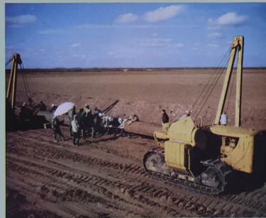
The desert draws vivid colour from pipe-laying activities
