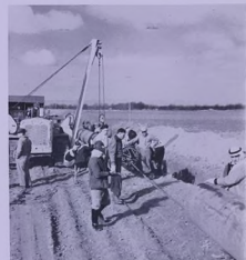
Top: surveyors are always first in the field. Middle: a back-acting shovel reaches the 466.4 signpost on the Kirkuk-Banias pipeline. Bottom: 30-inch pipe being aligned beside the ditch near T4 Pump Station
