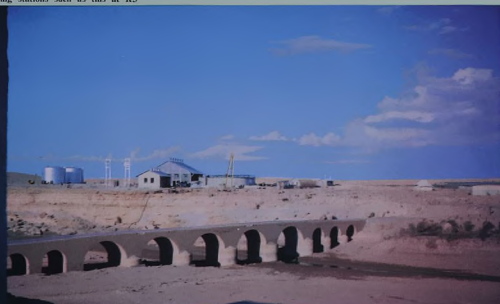
Water is supplied all along the line by wells or pumping stations such as this at K3
