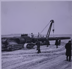
Left: a Buckeye Ditcher cuts part of the 556-mile 4 x 5-foot trench. Right: 30-inch pipe takes up a 15' bend like wax; pipe ends are bevelled before welding; a Mighly Anty, with trailer stowed, awaits its next 65-ton load of 30-inch pipe
