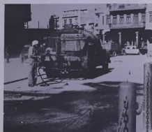
Road metalling works in progress in various areas of the Capital.
