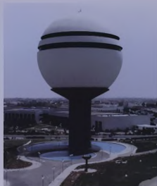
Al-Qassim Water Tower.
