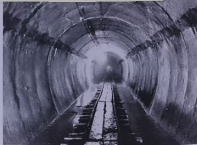
inside the Kuhrang tunnel
