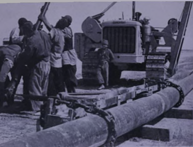
along the pipelines . . .
