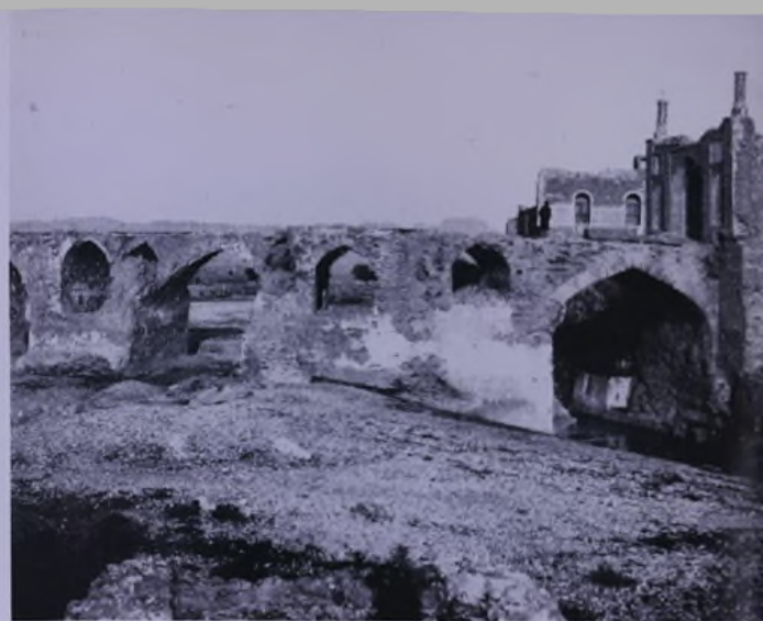
'Valerian's bridge' at Shushtar
