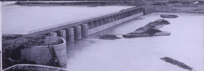
The Karkheh dam in Khuzistan
