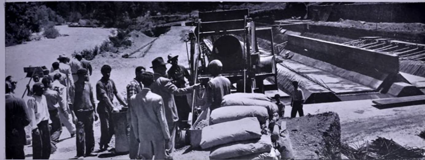
Water supply: construction of scheme for Teheran
