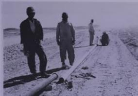
*Khalifa Suwaid with other members of the water gang connecting pipes which will carry drilling water to Rig 7 from a nearby water well.*
