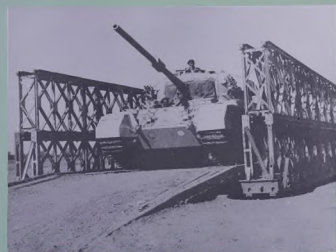
A tank crossing a military bridge built by the Engineering Battalion.
