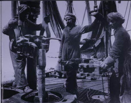
A Kuwaiti drilling crew at work
