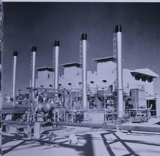
The sea-water distillation plant
