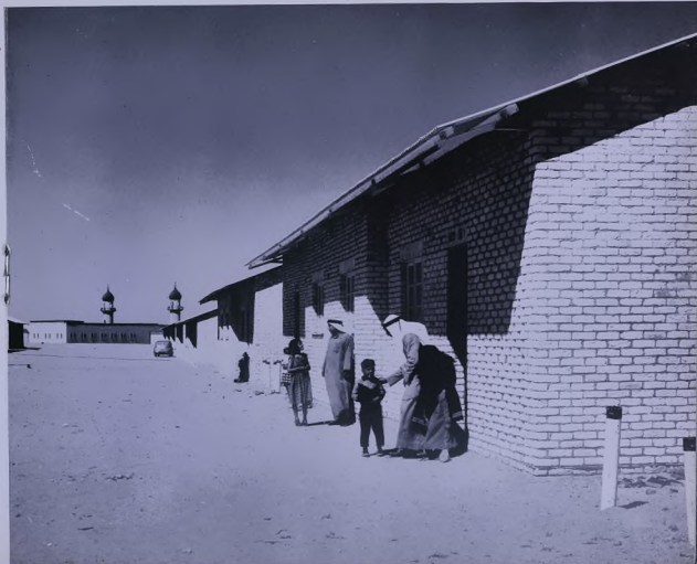
Housing for Company Arab employees, South Ahmadi
