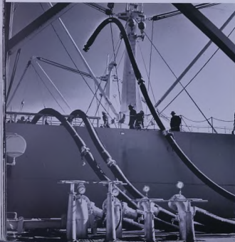
Loading in progress
