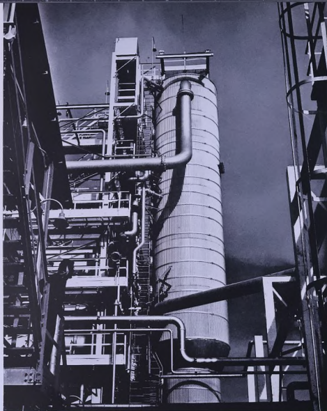
The refinery, Mina al Ahmadi
