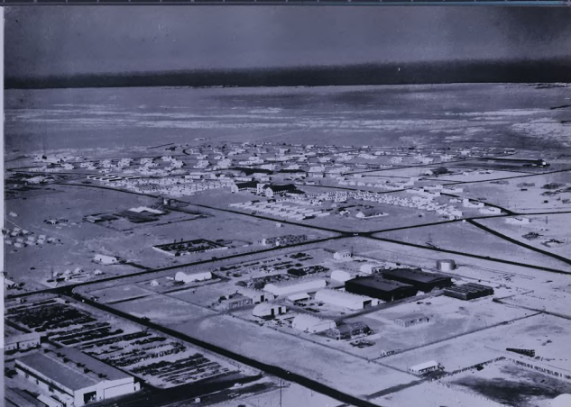
Industrial area and housing estates at Ahmadi, from the air
