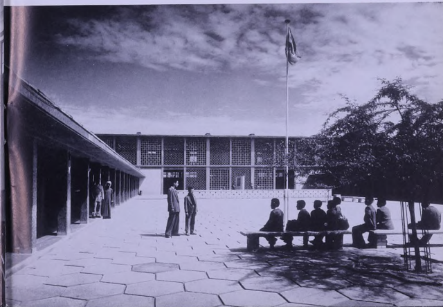
General view of a primary school in Kuwait
