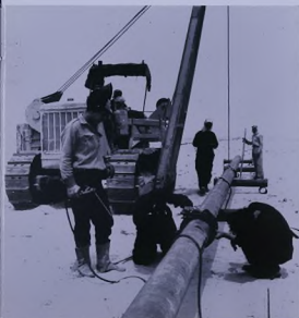
Laying a gas line to Kuwait Town
