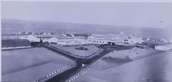
Kuwait Oil Company's hospital at Magwa
