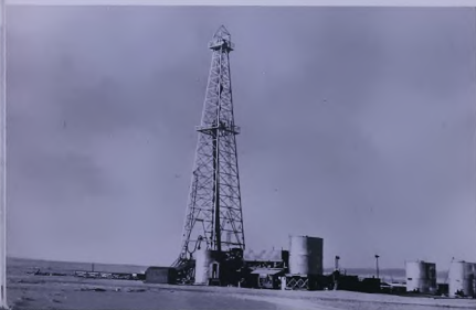
A drilling rig at Burgan
