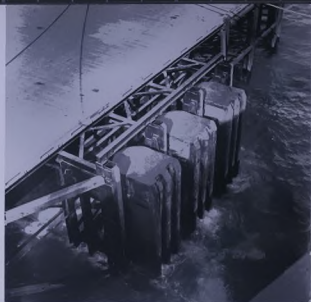
The Baker gravity fenders against which tankers are berthed
