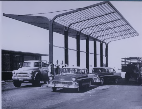
One of the major filling stations in Kuwait Town
